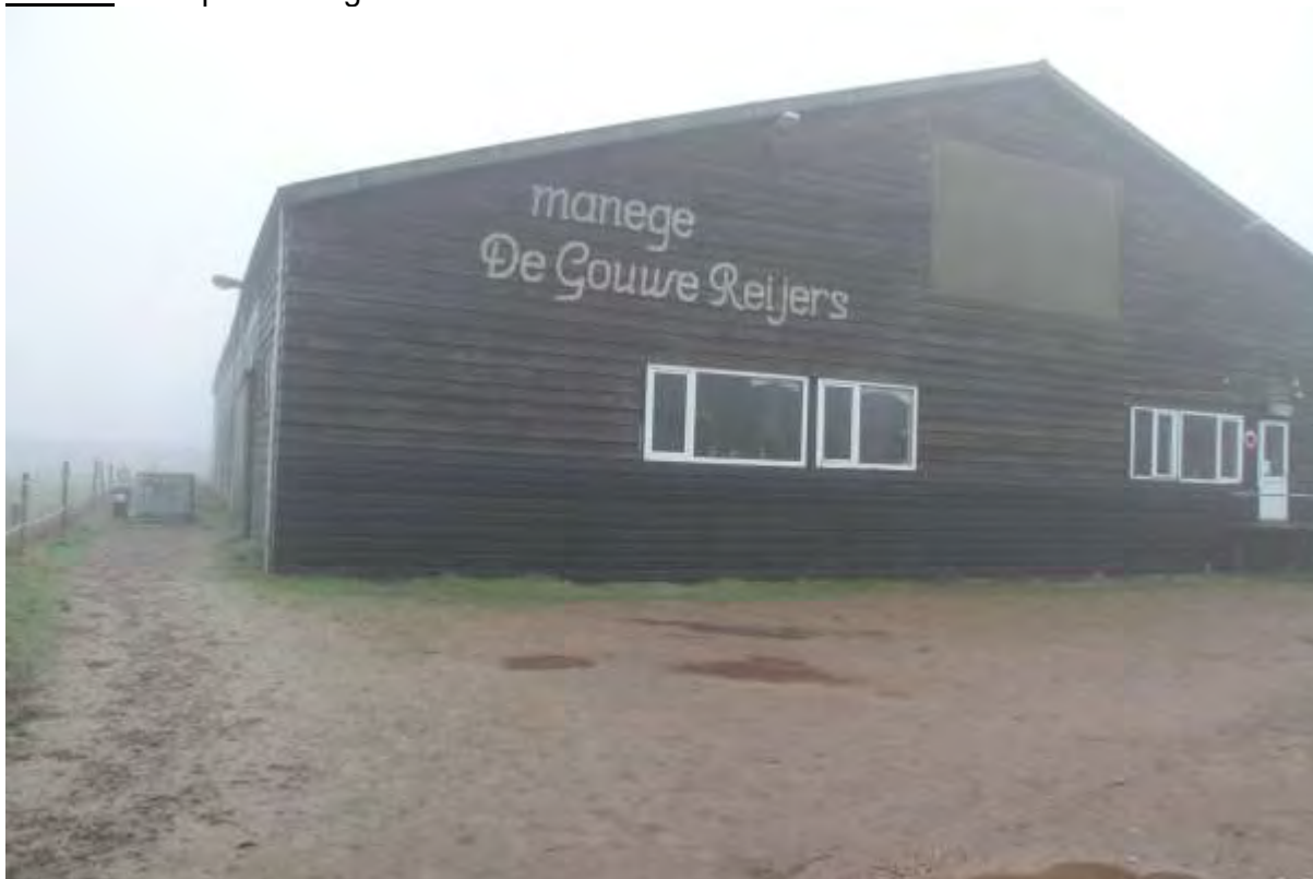
Foto 1. Te slopen manege.
